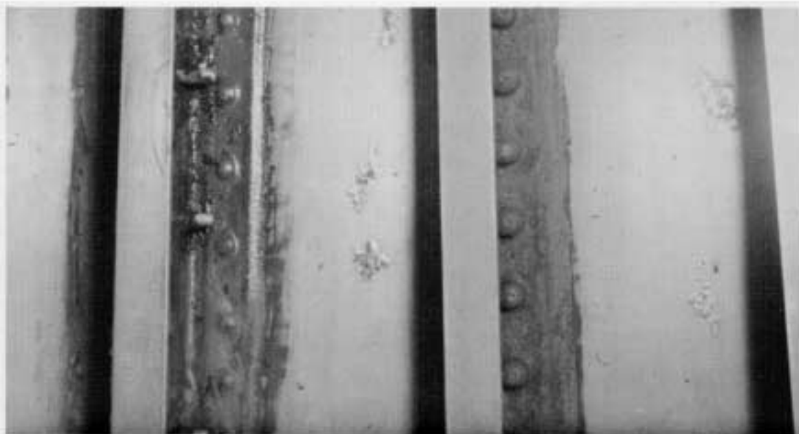
FIGURE 3. C-130 fuel tank after removal of the Buna-N shows the corrosion blisters and pockets.
