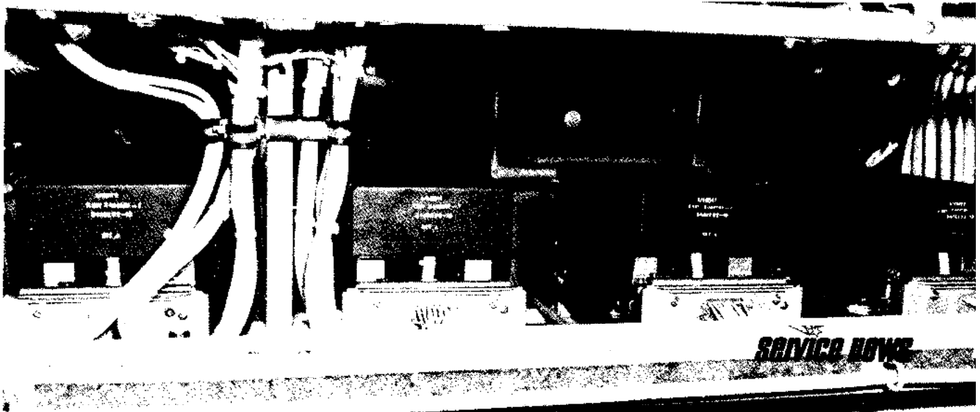
AC voltage regulators on the electrical control and supply rack just forward of the 245 bulkhead.
