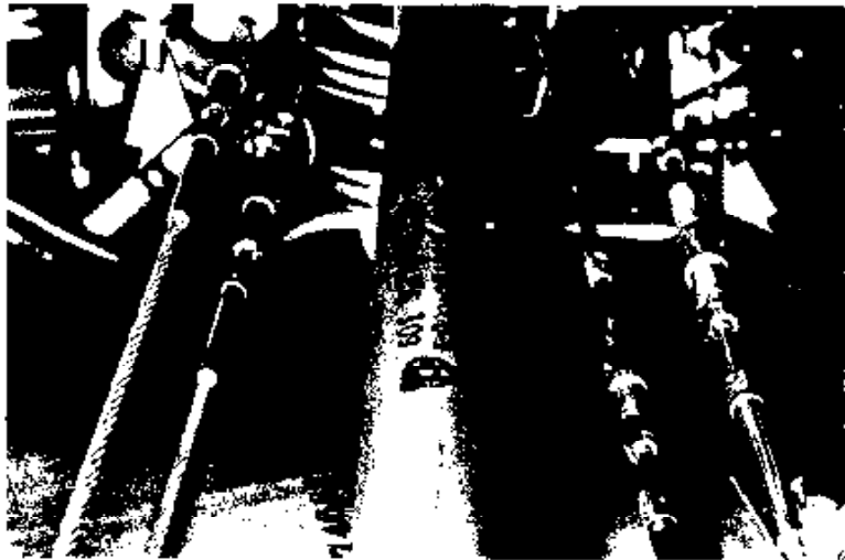
Outboard lower control cable turnbuckles used to adjust condition lever preload.
