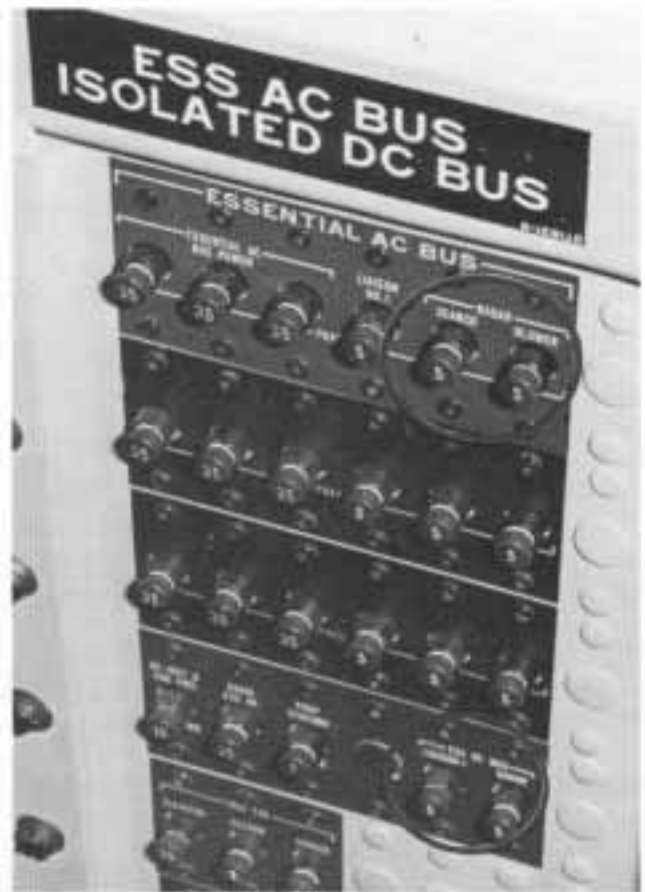
Circuit breakers for the APQ-122 radar.
