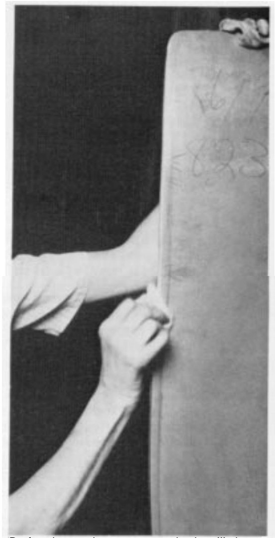
Performing a dye penetrant check will determine if all corrosion cracks have been removed.
