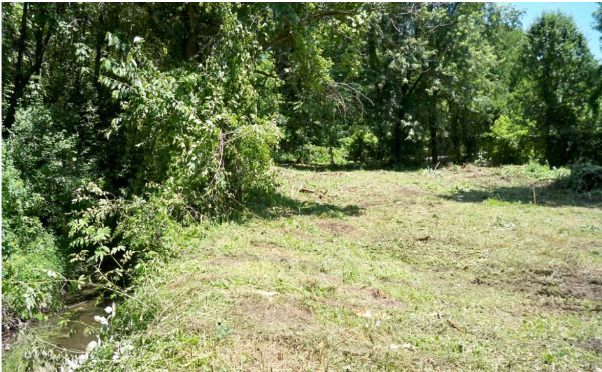
Photo #4: South Zone partially cleared
