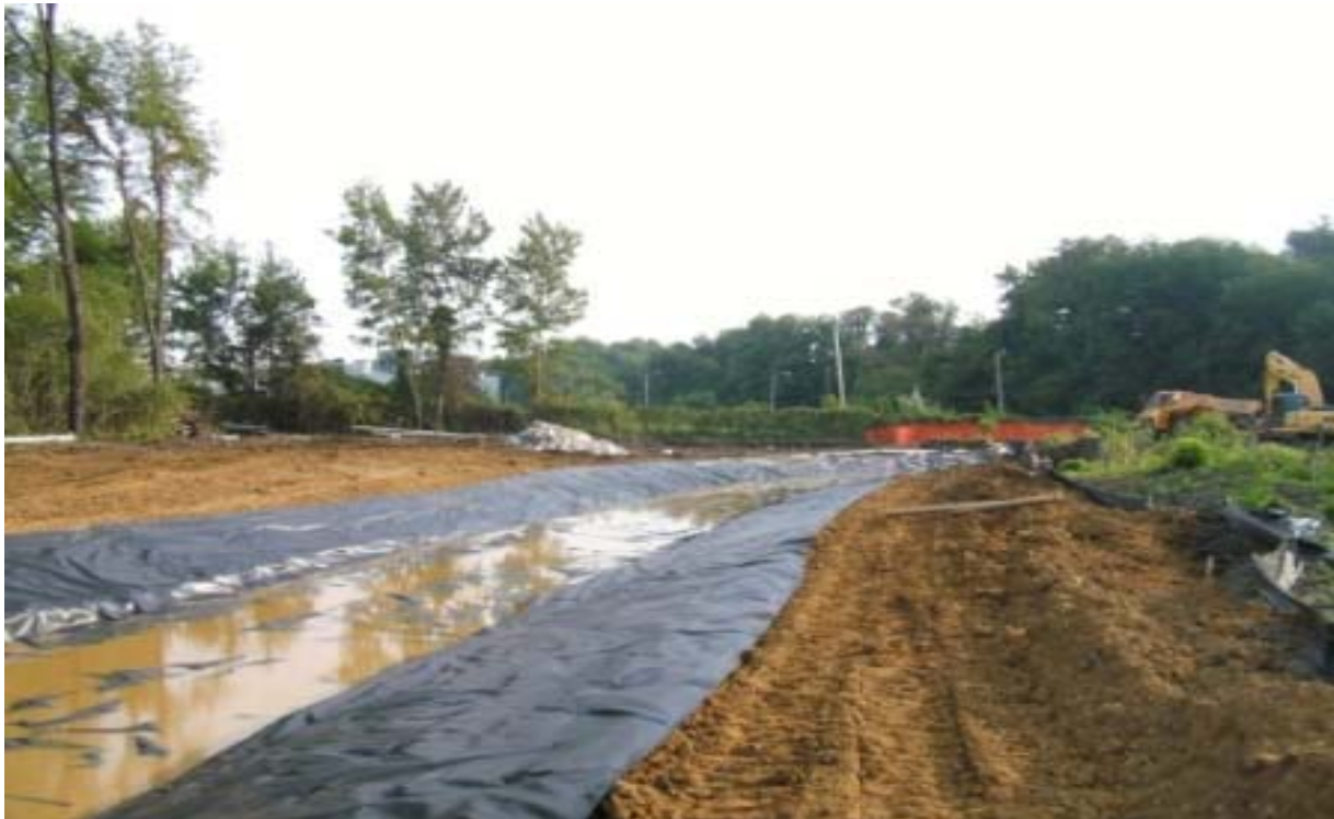
Photo #18: Lined bypass channel constructed in the South Zone
