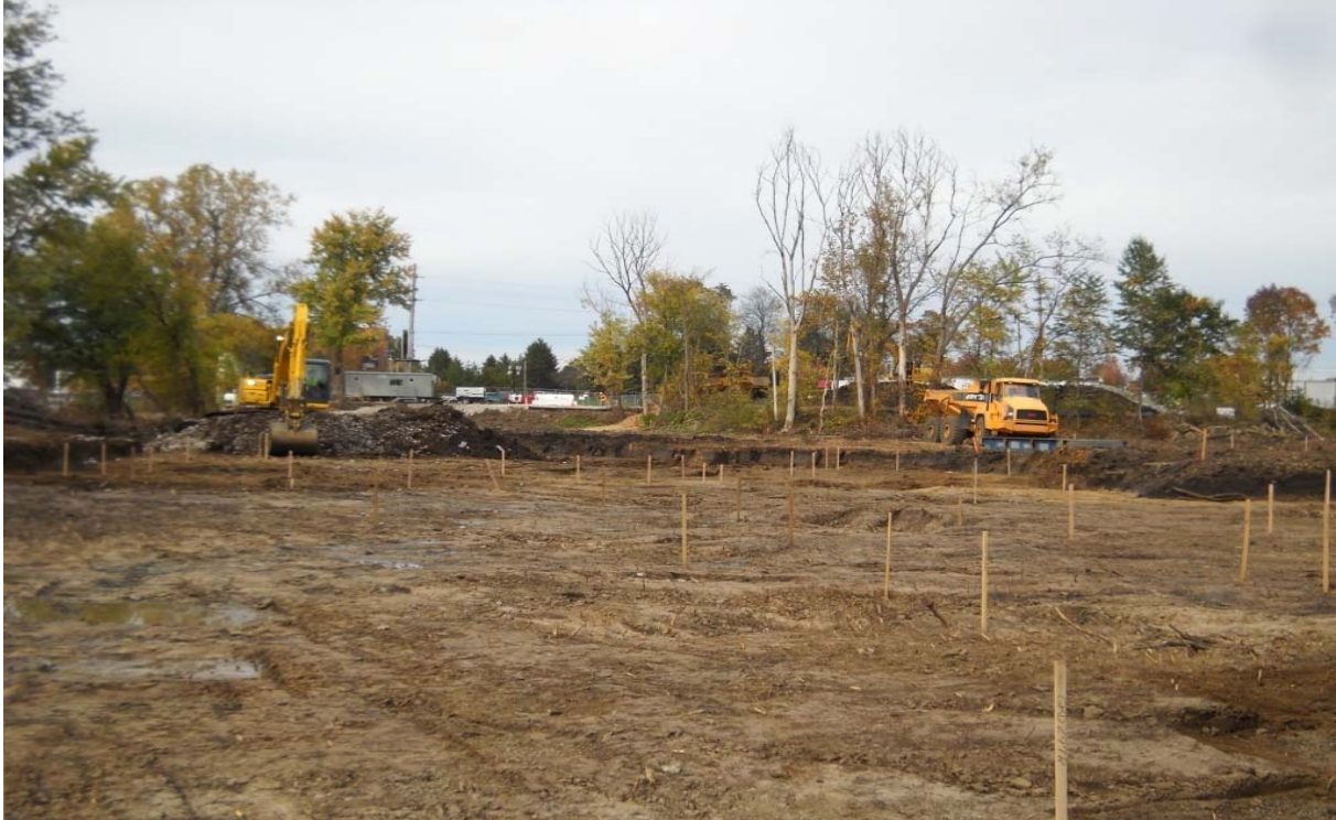
Photo #27: North Zone excavation with verification sample locations staked
