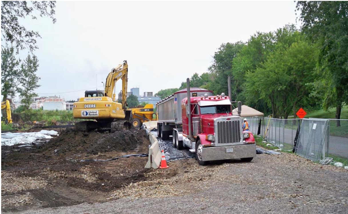
Photo #22: South Zone truck loading operations
