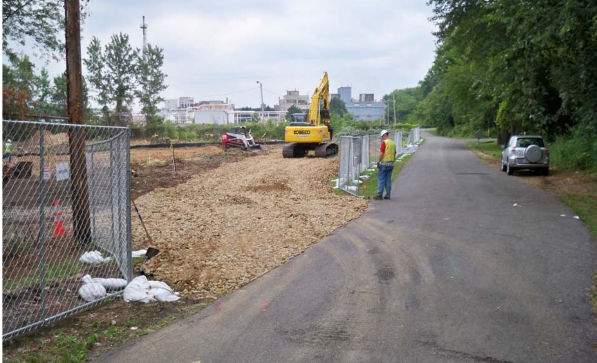
Photo #9: South Zone construction entrance
