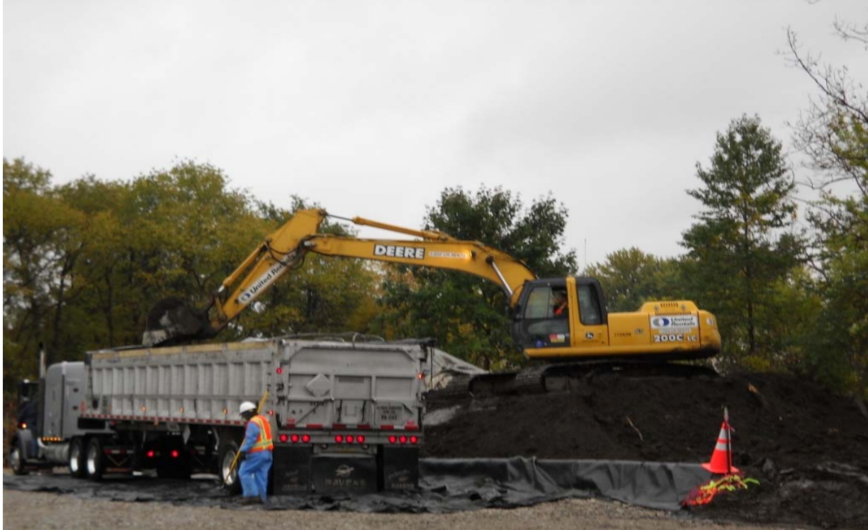
Photo #29: North Staging Area truck loading operations
