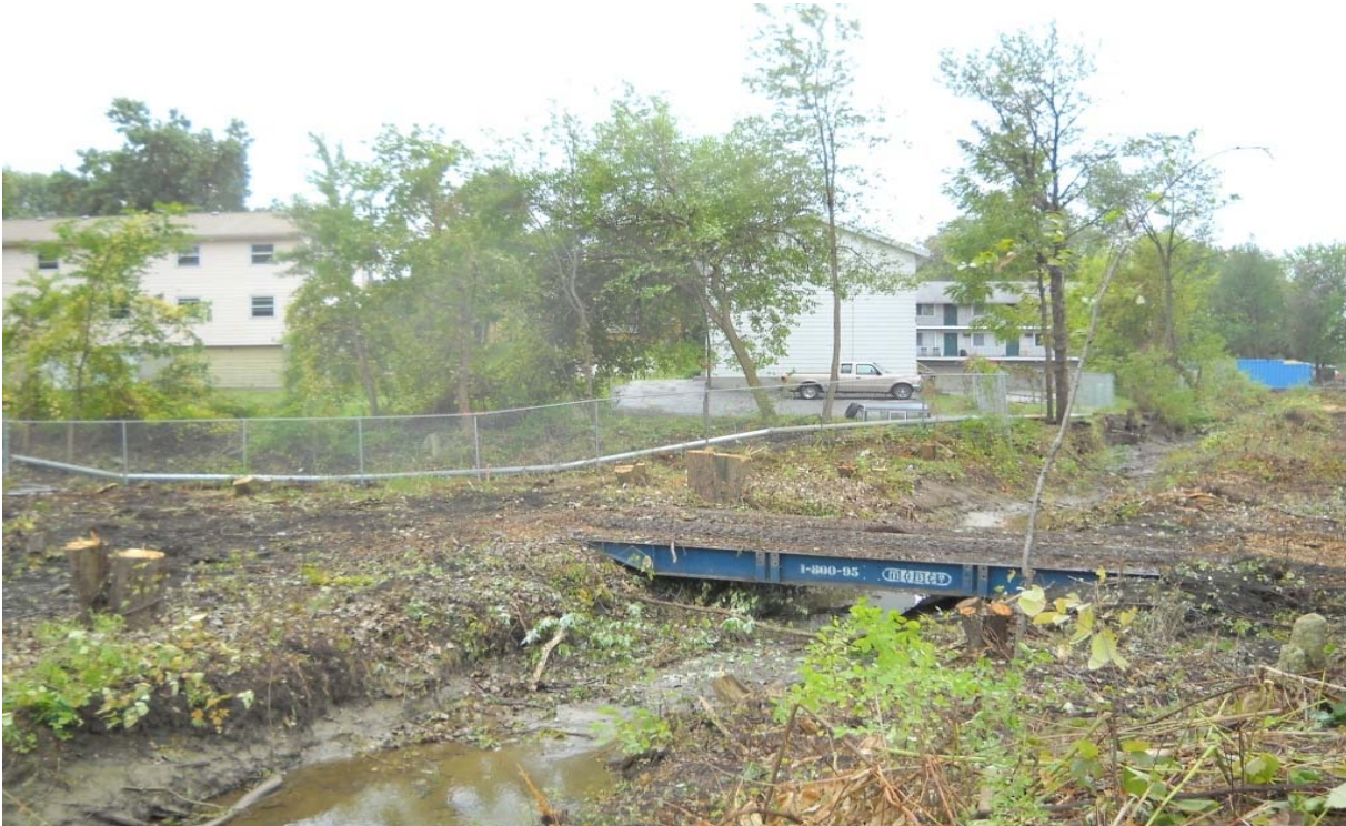
Photo #14: Temporary bridge used for stream crossing
