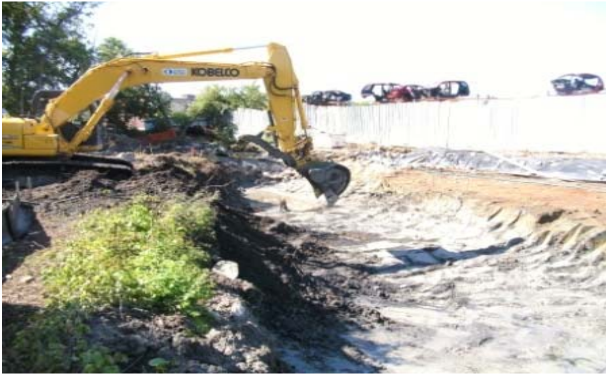
Photo #21: South Zone channel excavation
