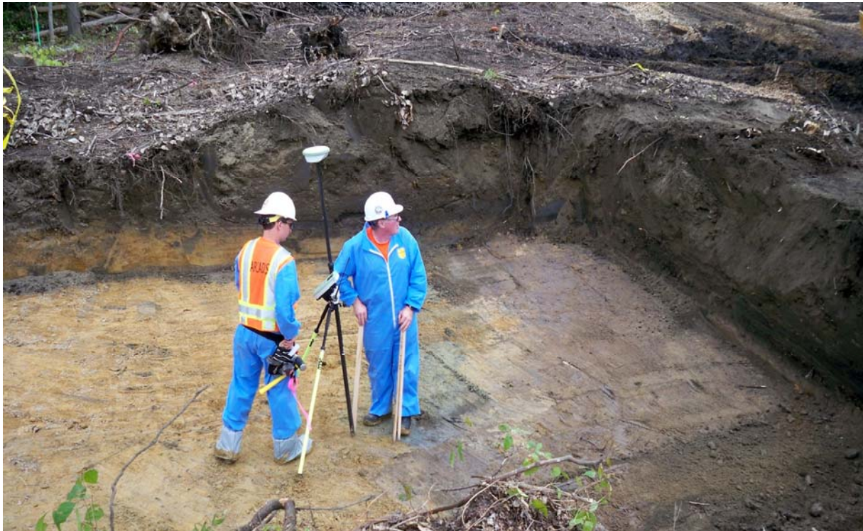
Photo #24: Using GPS to locate verification samples within an excavated grid
