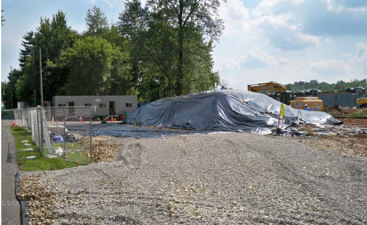
Photo #23: South Zone soil stockpile secured with plastic sheeting
