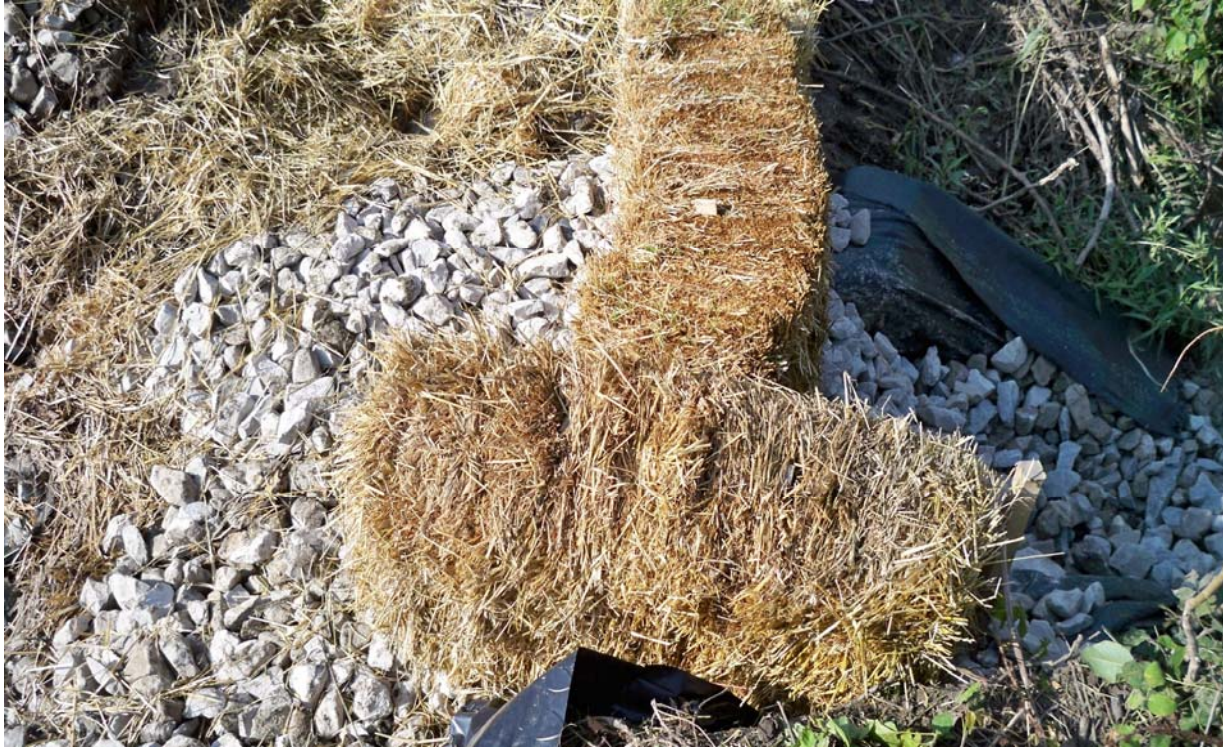
Photo #13: Stone check dam with hay bales installed within channel
