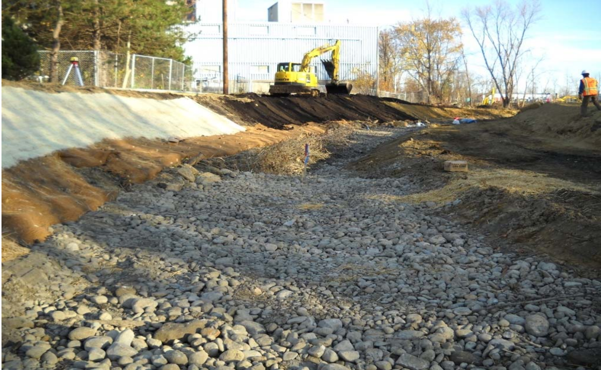
Photo #31: Middle Zone undergoing restoration
