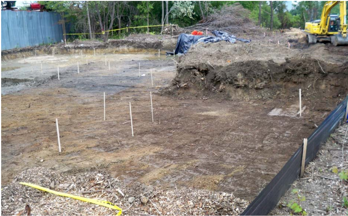
Photo #25: South Zone excavated grids with verification sample locations staked
