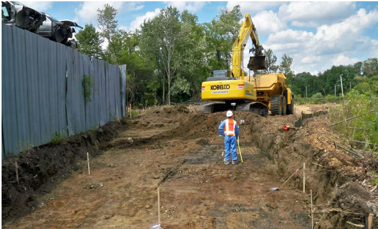
Photo #20: South Zone soil excavation and loading
