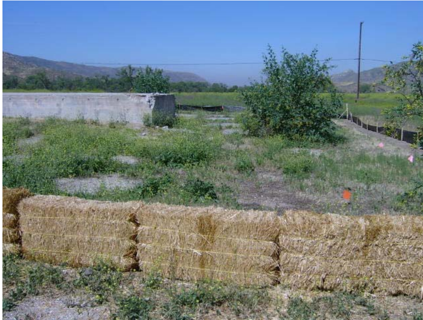
Photo 29: Use of silt fence and straw bales with attached silt fence fabric used to confine and exclude SKR while trapping activities were being conducted. Once an area was fully trapped, removal action commenced. After removal was complete silt fence and straw bales were removed and ground was leveled. (Note use of pin flags to denote burrow locations)
