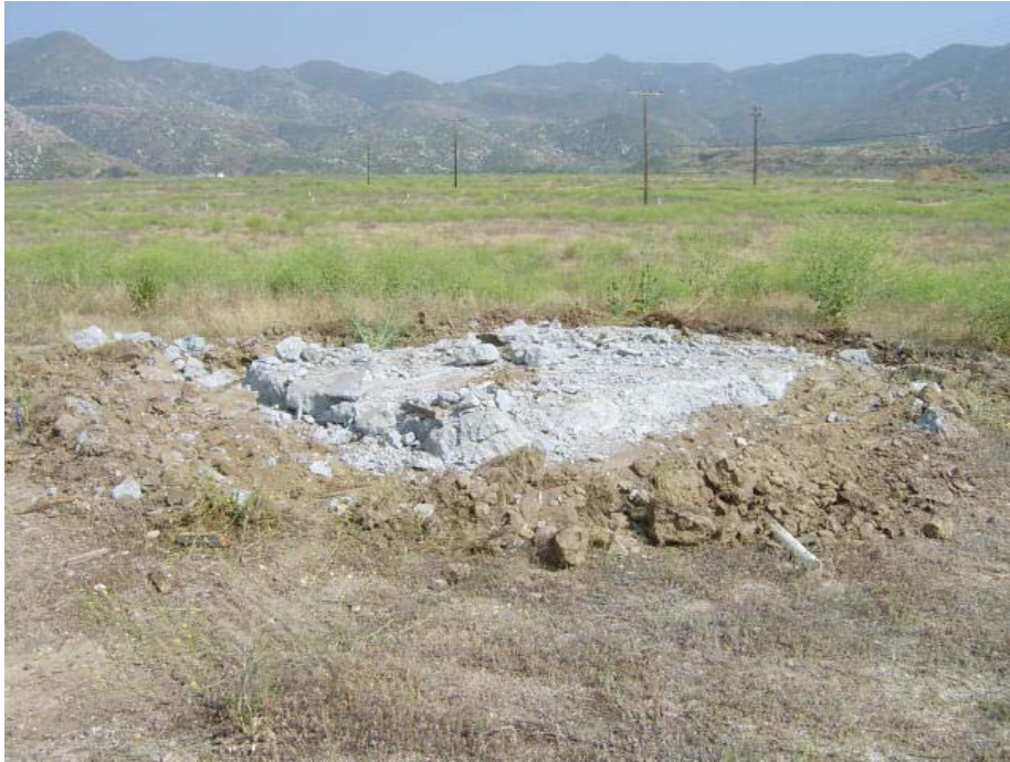
Photo 7: Offset Area 1 – Removal of concrete pad located west of Building 315
