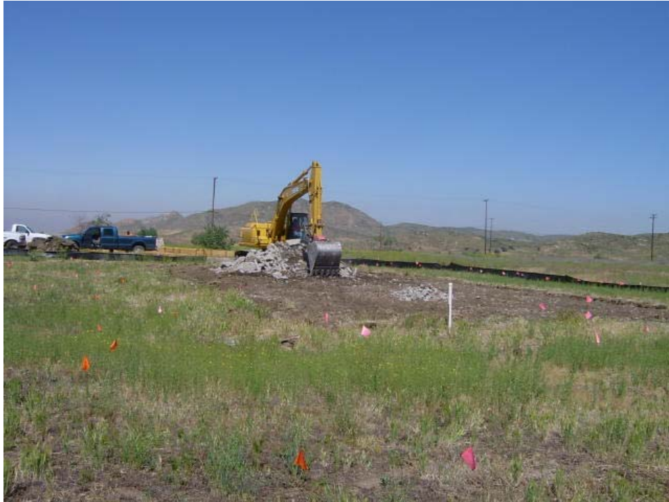
Photo 13: Offset Area 3 – Removal of former chemical storage building pad. (Note use of pin flags to denote burrow locations)
