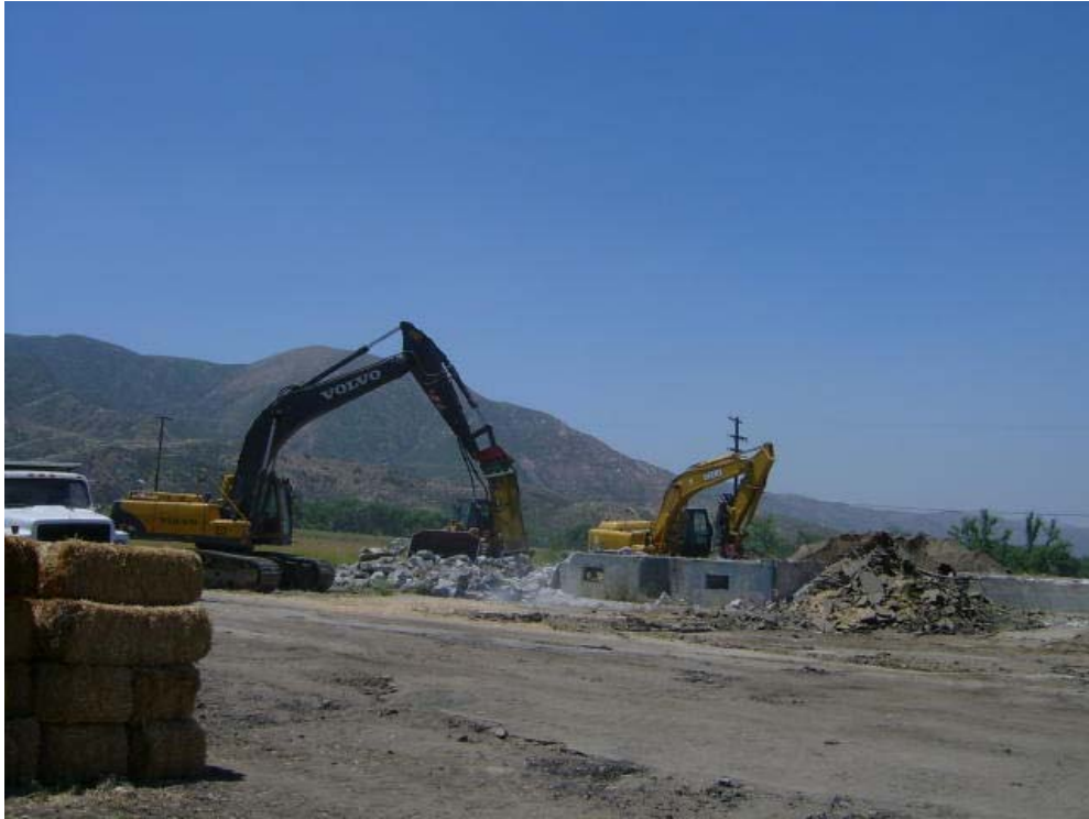
Photo 9: Offset Area 2 – Removal of former fuel slurry station
