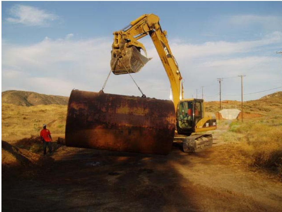
Photo 4: Exhibit H Item 7 – Removal of water storage tank above Building 304
