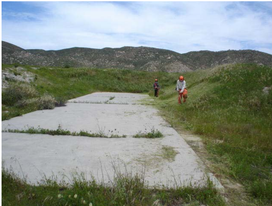
Photo 24: Vegetation clearance and mowing activities using hand carried weed cutting equipment.
