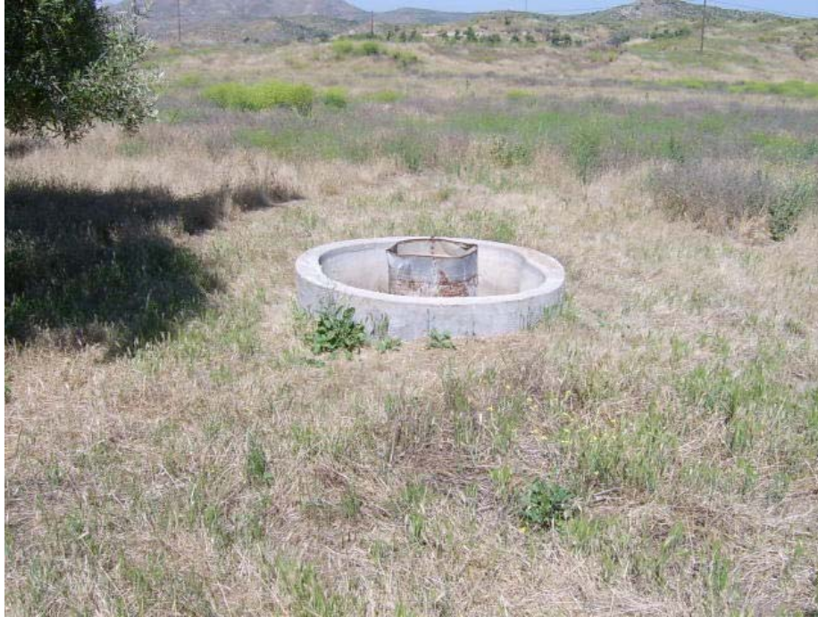
Photo 1: Exhibit H Item 4 – Circular concrete structure before removal
