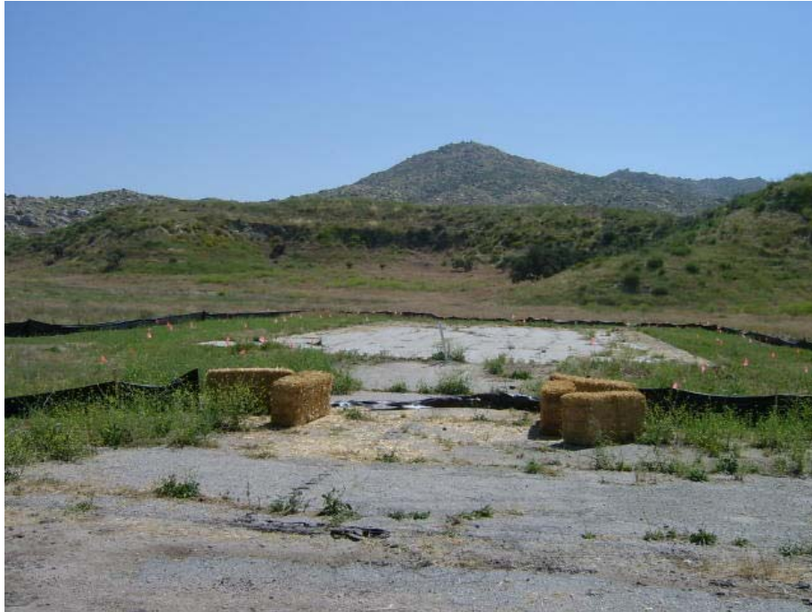
Photo 11: Offset Area 3 – Removal of former chemical storage building pad. (Note silt fence and straw bales used to exclude and contain SKR while conducting trapping activities)
