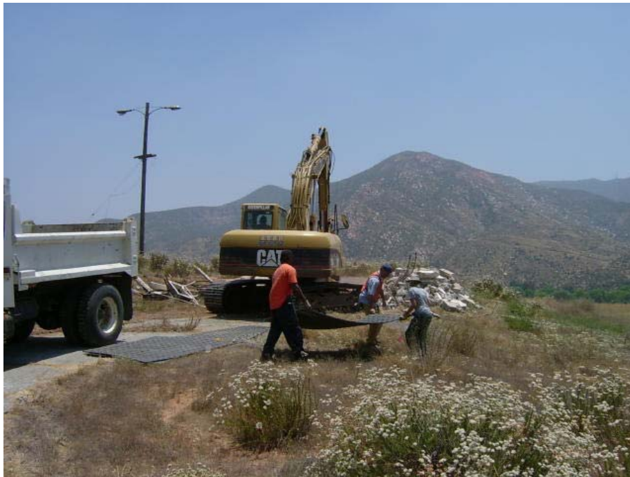
Photo 26: Large (4' x8') load bearing mats used for SKR avoidance and protection
