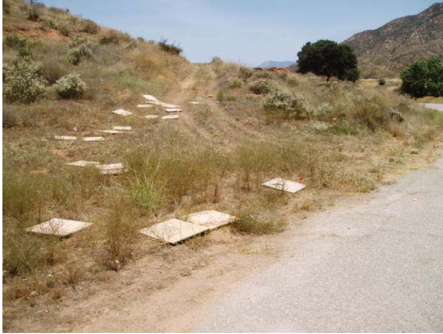
Photo 25: Small (2' x2') load bearing mats used for SKR avoidance and protection.
