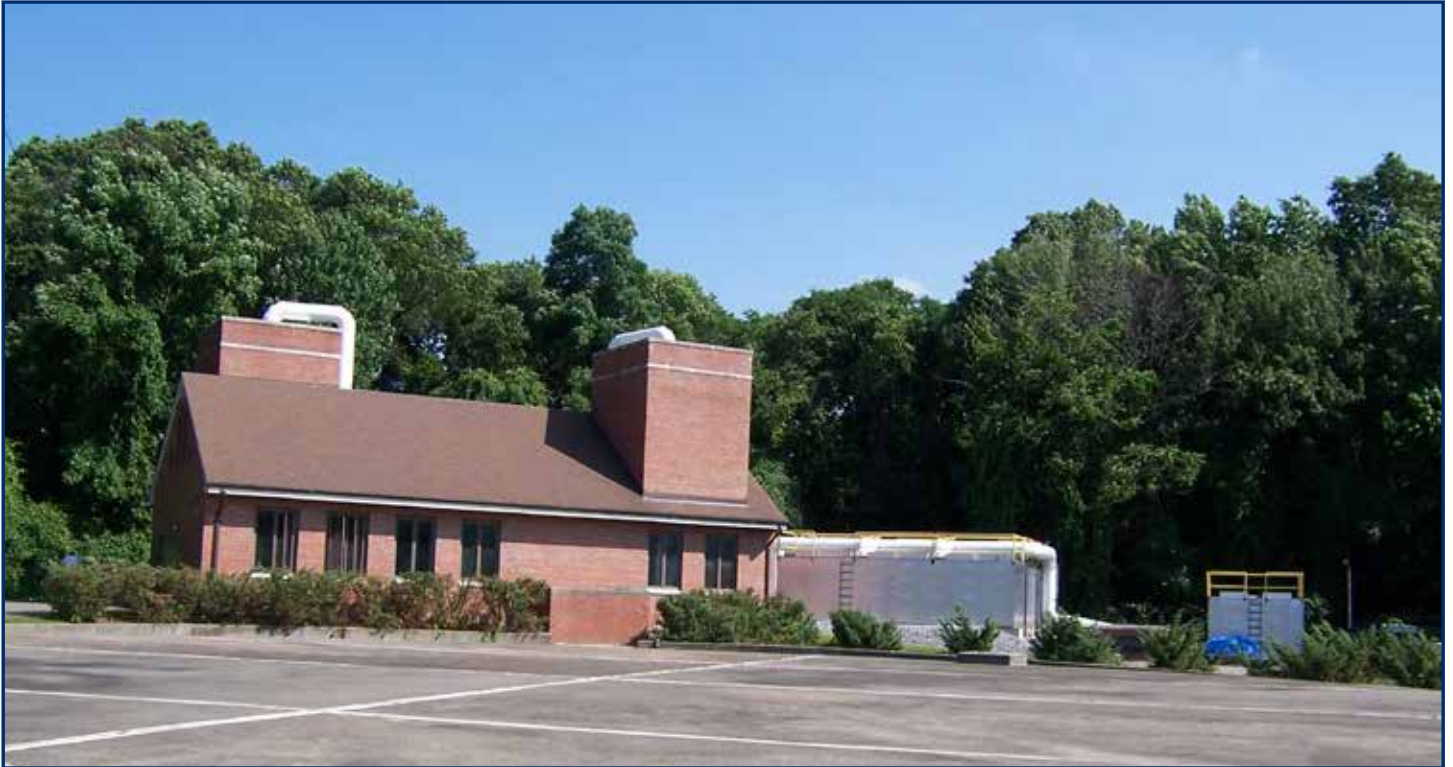
Off-Site (OU-2) Groundwater Treatment System
