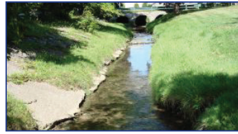
Slumped flagstone – before restoration
