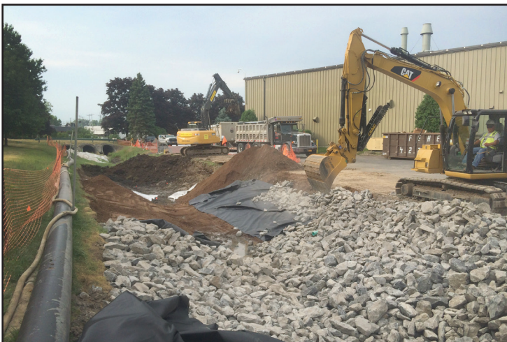
Simultaneous brook restoration (foreground) and remedial excavation (background).
