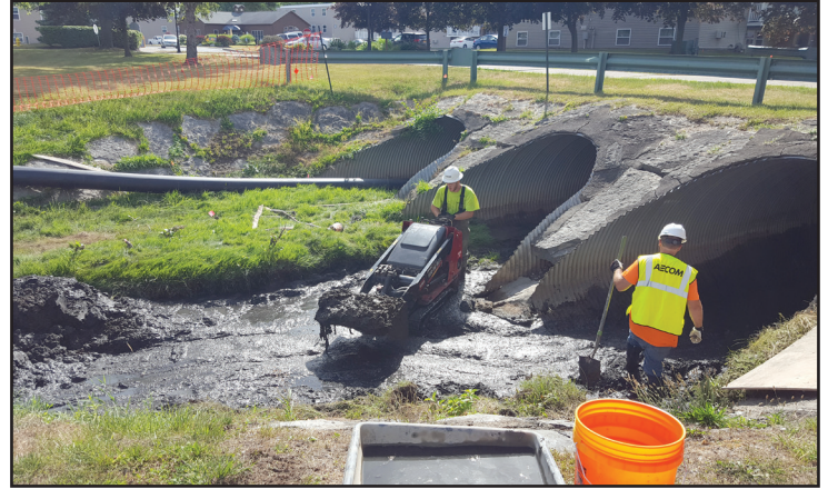
Sediment removal from culverts beneath Town Garden Drive.
