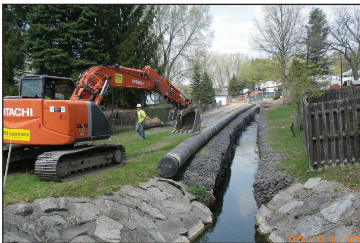
Installation of bypass pump piping near Brookview Lane culverts.
