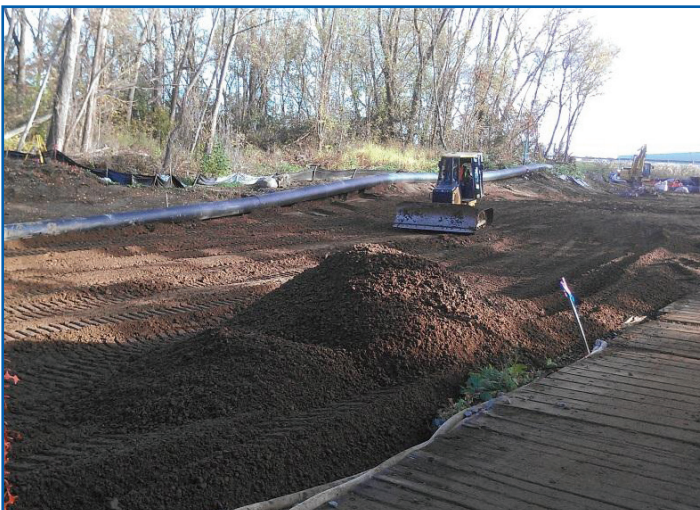
Placing general backfill near middle wetland/pond area.
