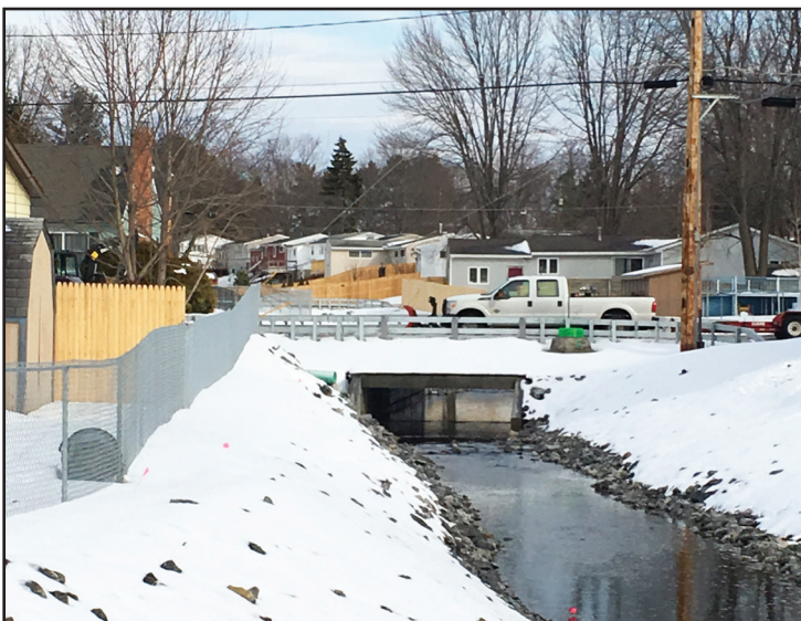
View from Floradale Road looking upstream at the new concrete culvert at Sunflower Drive, the restored brook and new residential fencing.
