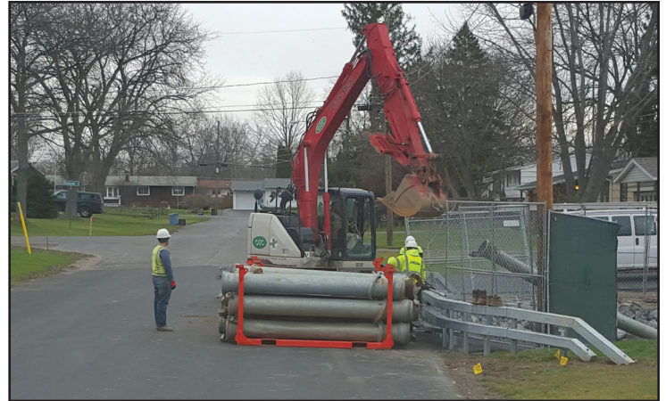
Removal of bypass pump piping at the completed Brookview Lane culvert.
