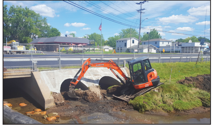
Removal of brook sediment from the culverts underneath Old Liverpool Road.
