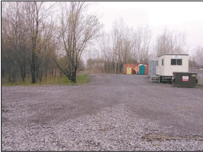
2016 construction staging area off of Old Liverpool Road.
