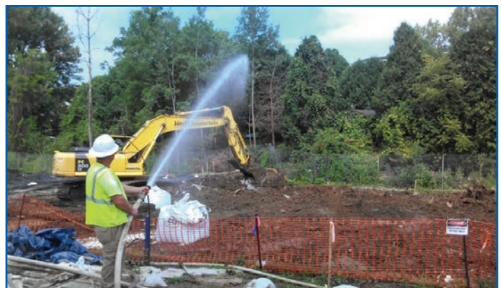
Spraying to control dust during excavation activities.
