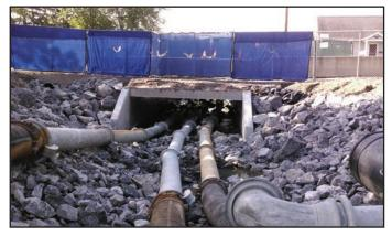
Bypass pump piping running through the new concrete box culvert underneath Brookview Lane.
