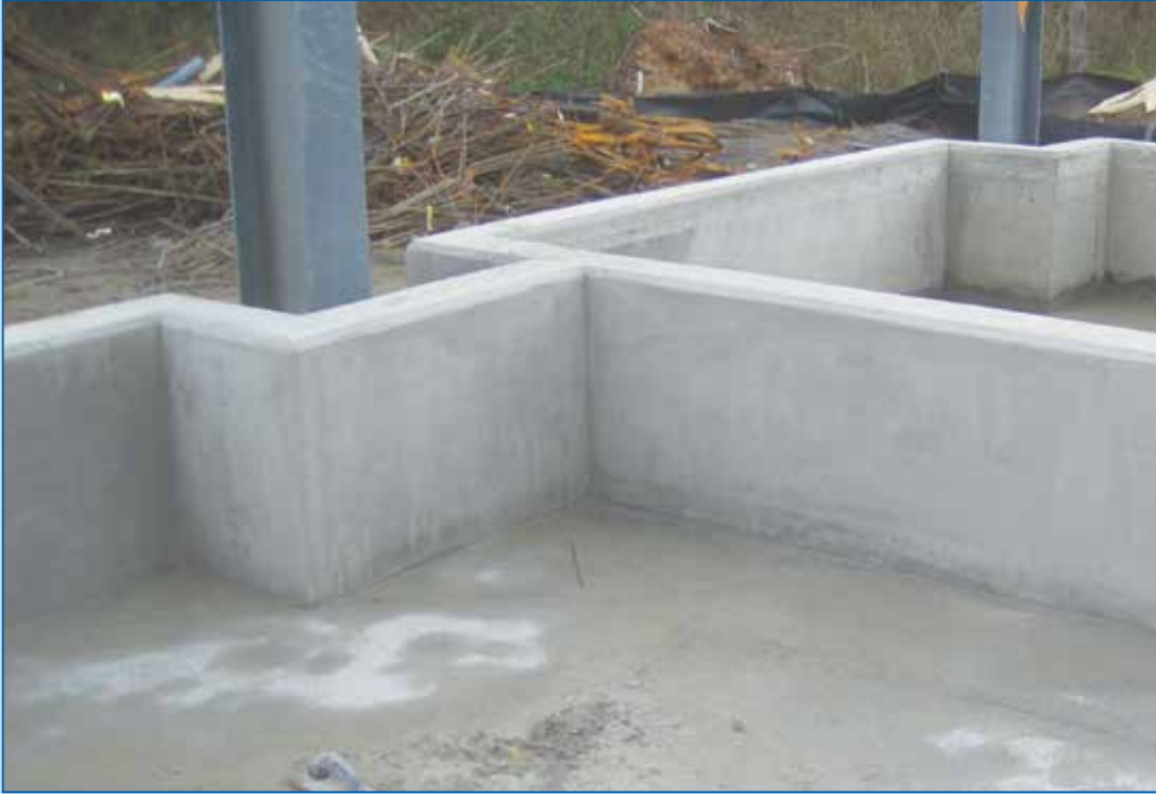
A hardener and sealant were applied to finish concrete floors and containment walls.
