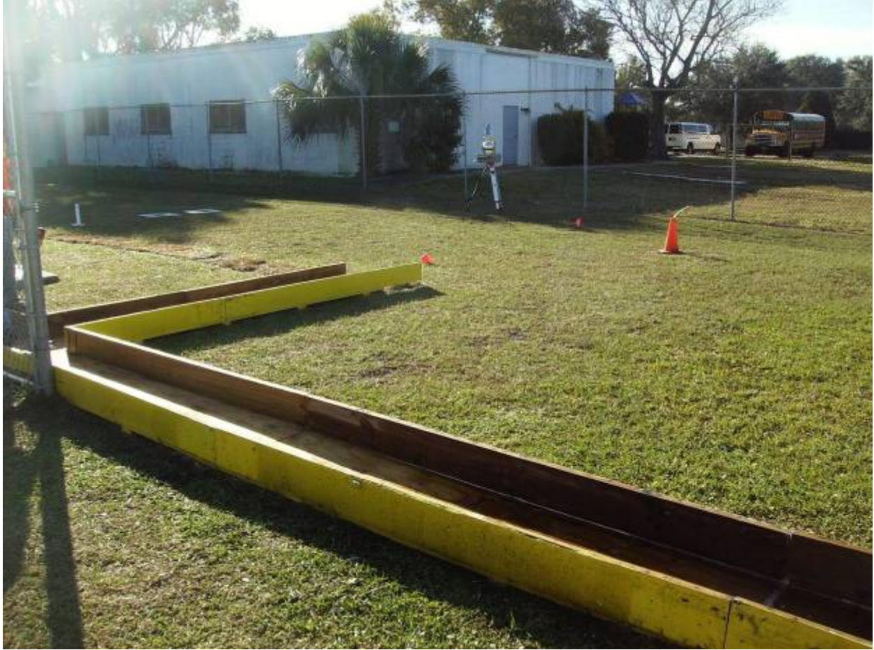
ISR System Containment Tray Demolition
