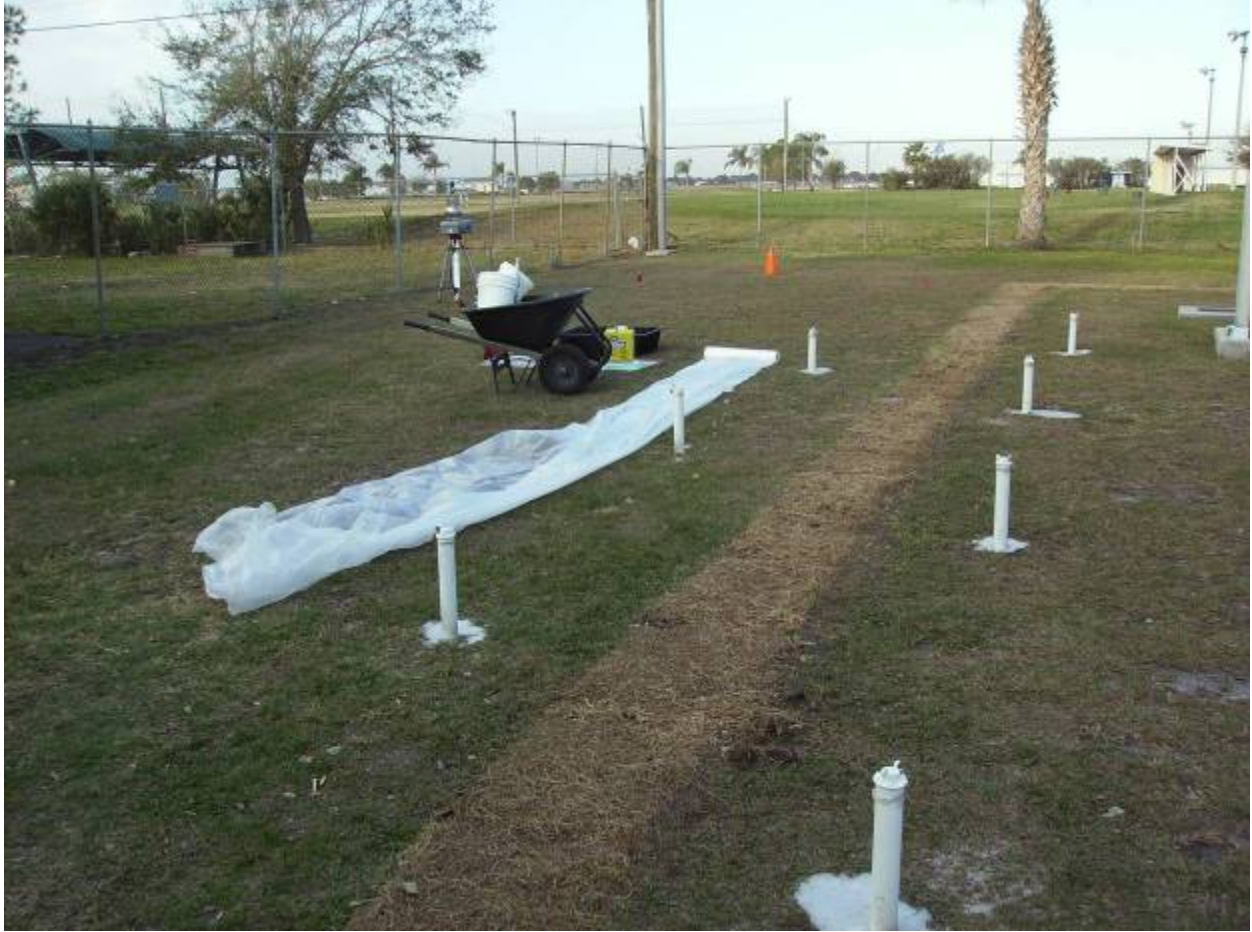
Preparation for ISR System Well Abandonment
