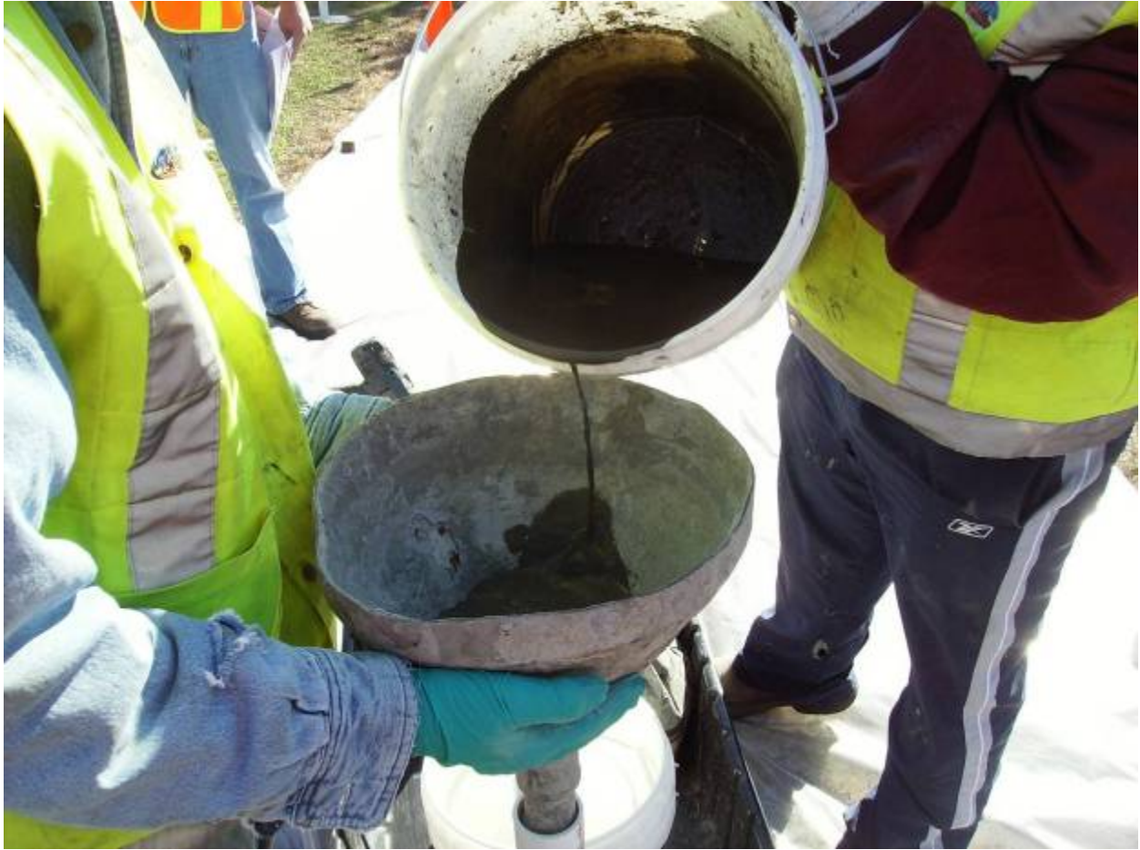
ISR System Well Abandonment
