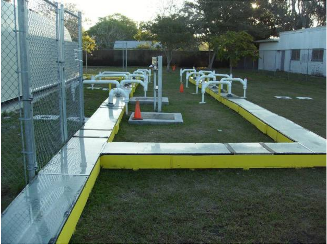
ISR System Pre-Demolition
