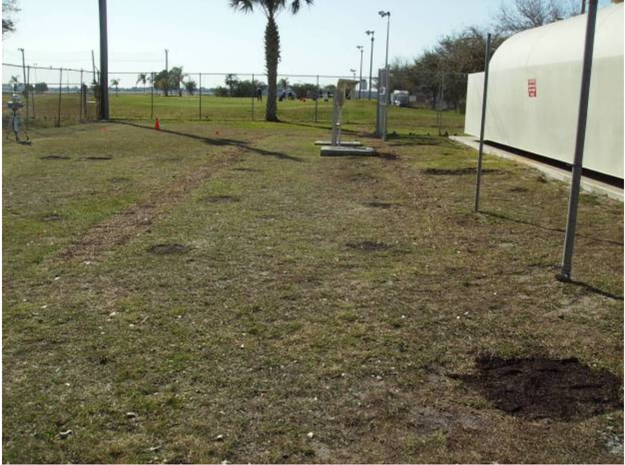
ISR System Demolition Site Restoration
