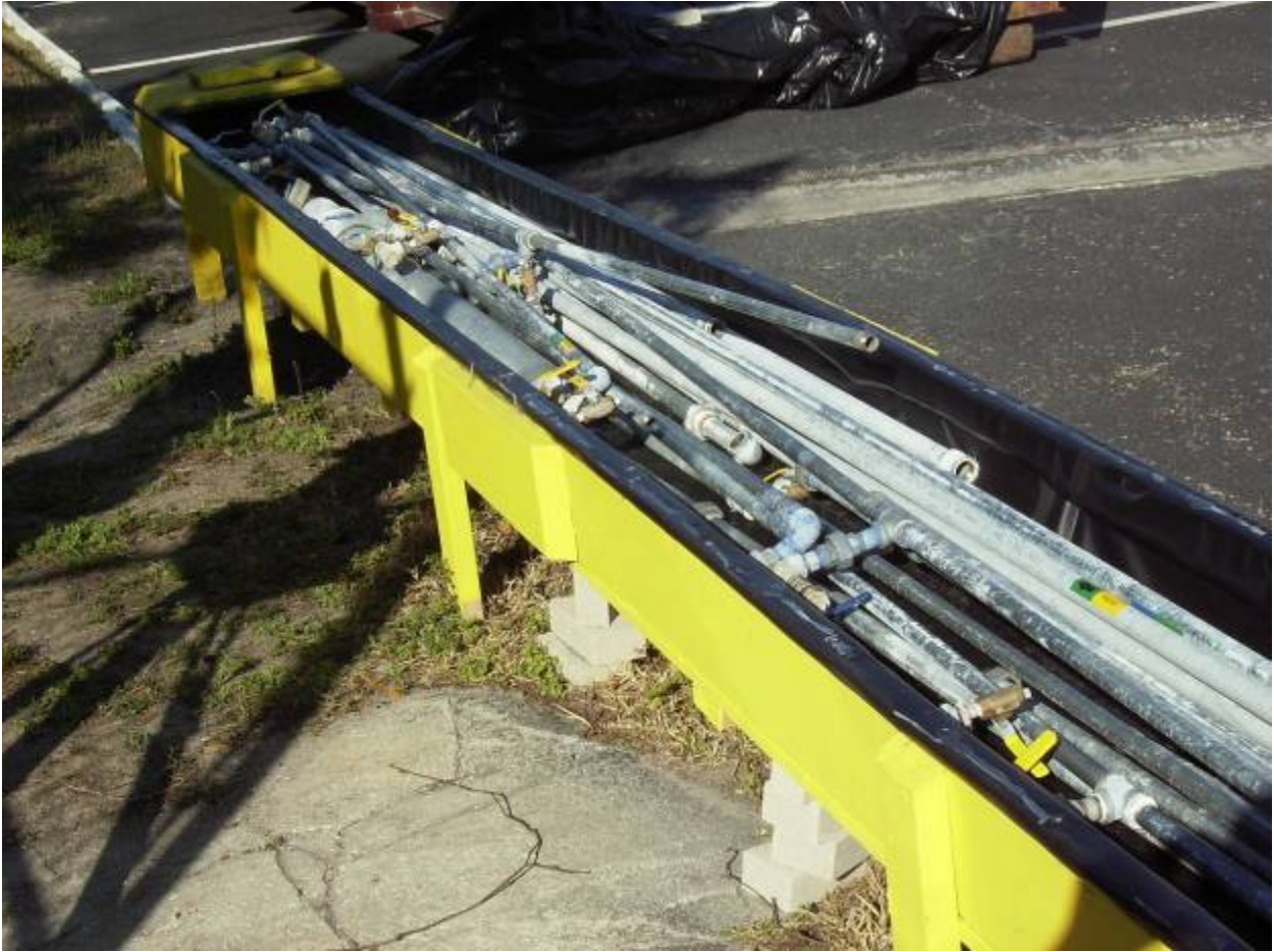
Steel Pipe from ISR System Staged for Off-Site Recycling
